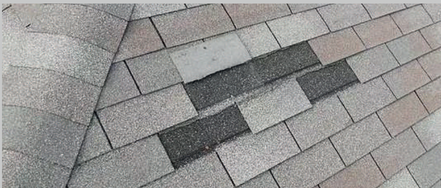
MISSING SHINGLES
